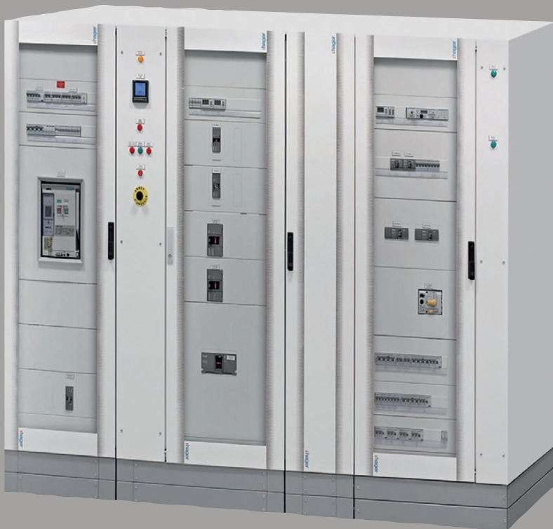
Switchboard for electrical distribution.
